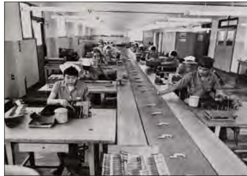
Conveyor-belt line during the 1960s
